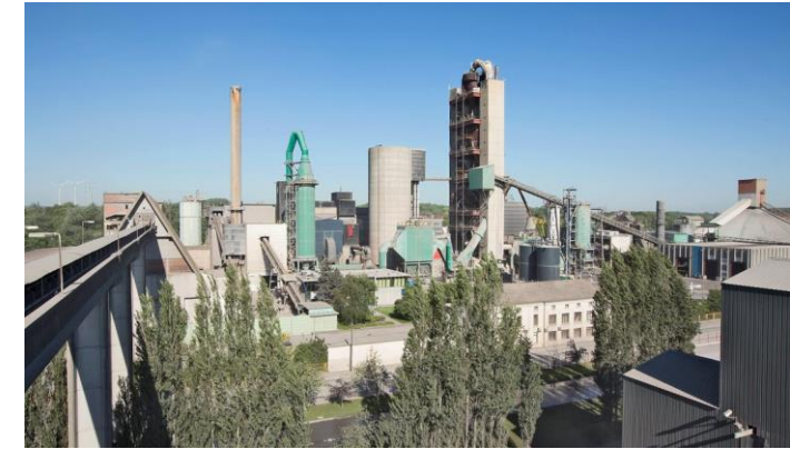
Heidelberg Materials to build one-of-a-kind hybrid carbon capture unit at its Belgian Antwerp cement plant
